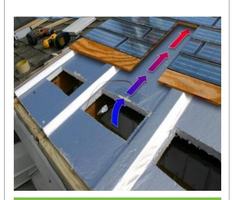
Sample advanced roof design applied to BIPV to be evaluated (50% reduction of roof thermal load)
