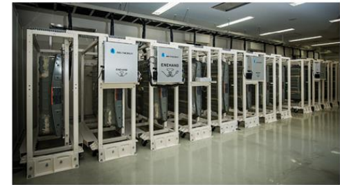
Large electrical energy storage facility Capacity: about 400kWh; Power: 250kW
