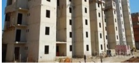
U \sim 3.5 \text{ W/m}^2\text{K} Monolithic concrete wall
