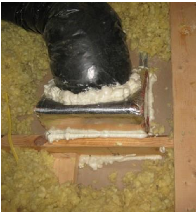
Sealing the connection
