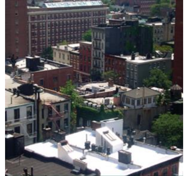
White reflective coating for cool roofs in New York, USA
