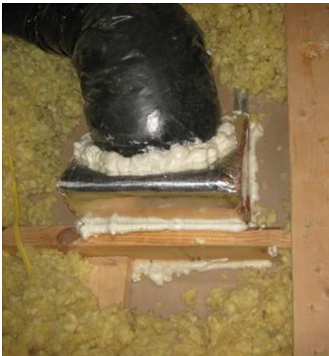
Sealing the connection
