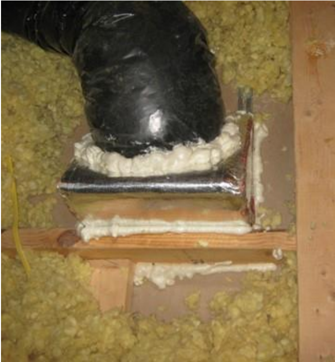
Sealing the connection
