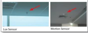
Lux sensor installed to monitor the illuminance level of the room, which will turn off automatically the artificial lighting within natural lighting area if the room illuminance more than 300 lux. Therefore it reduce energy consumption of artificial lighting.
