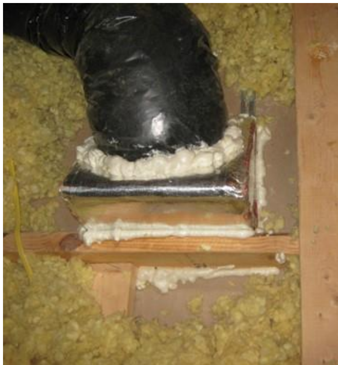
Sealing the connection
