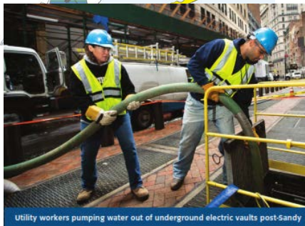
Utility workers pumping water out of underground electric vaults post-Sandy
