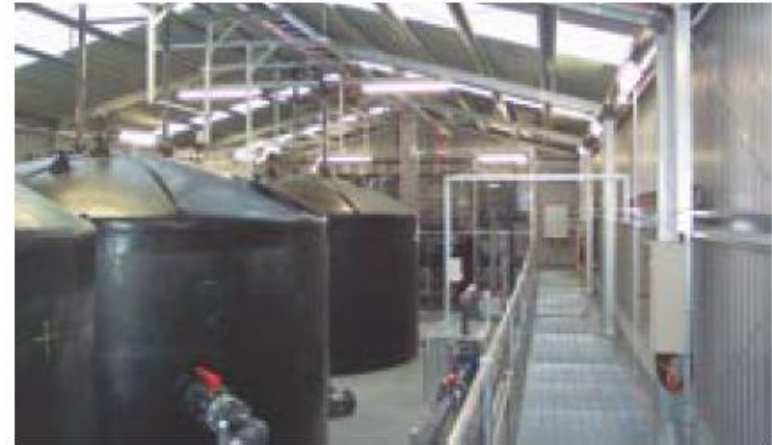
Vanadium Redox Battery System with the tanks containing electrolyte in the foreground and a bank of cell stacks at the far end of the building.
