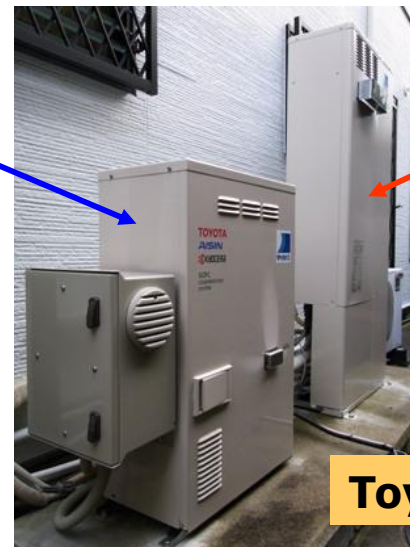
SOFC unit 0.7kW
