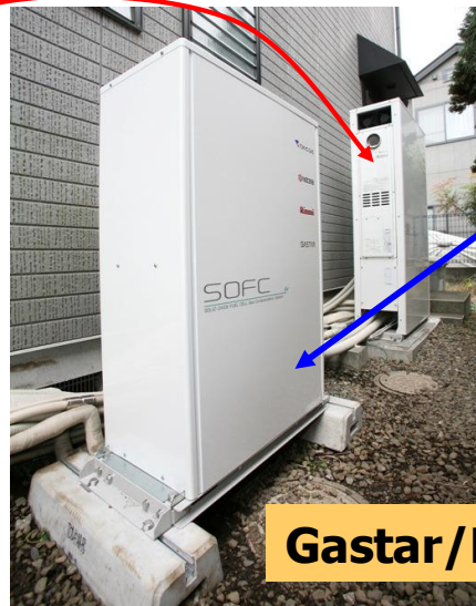
SOFC unit 0.7kW
