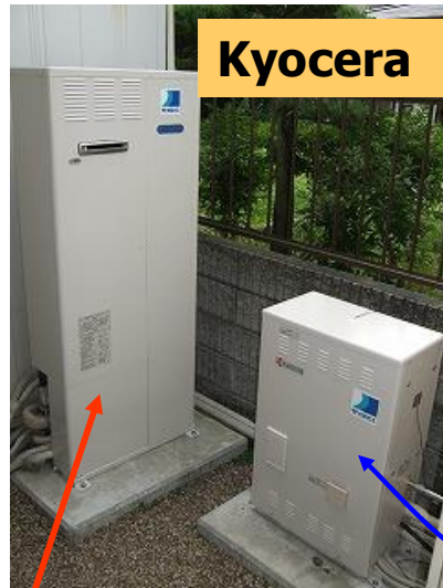
Hot Water Tank unit
