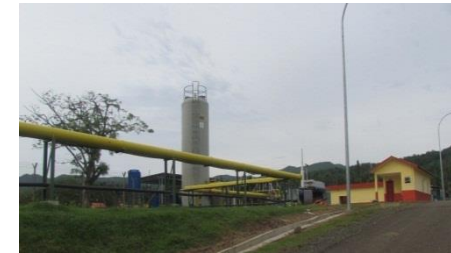
BIOGAS CAPTURED PIPING TO BIOSCRUBBER
