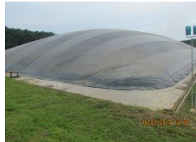
ANAEROBICS DIGESTER
