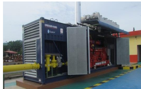
GAS ENGINE FOR ELECTRICITY GENERATION
