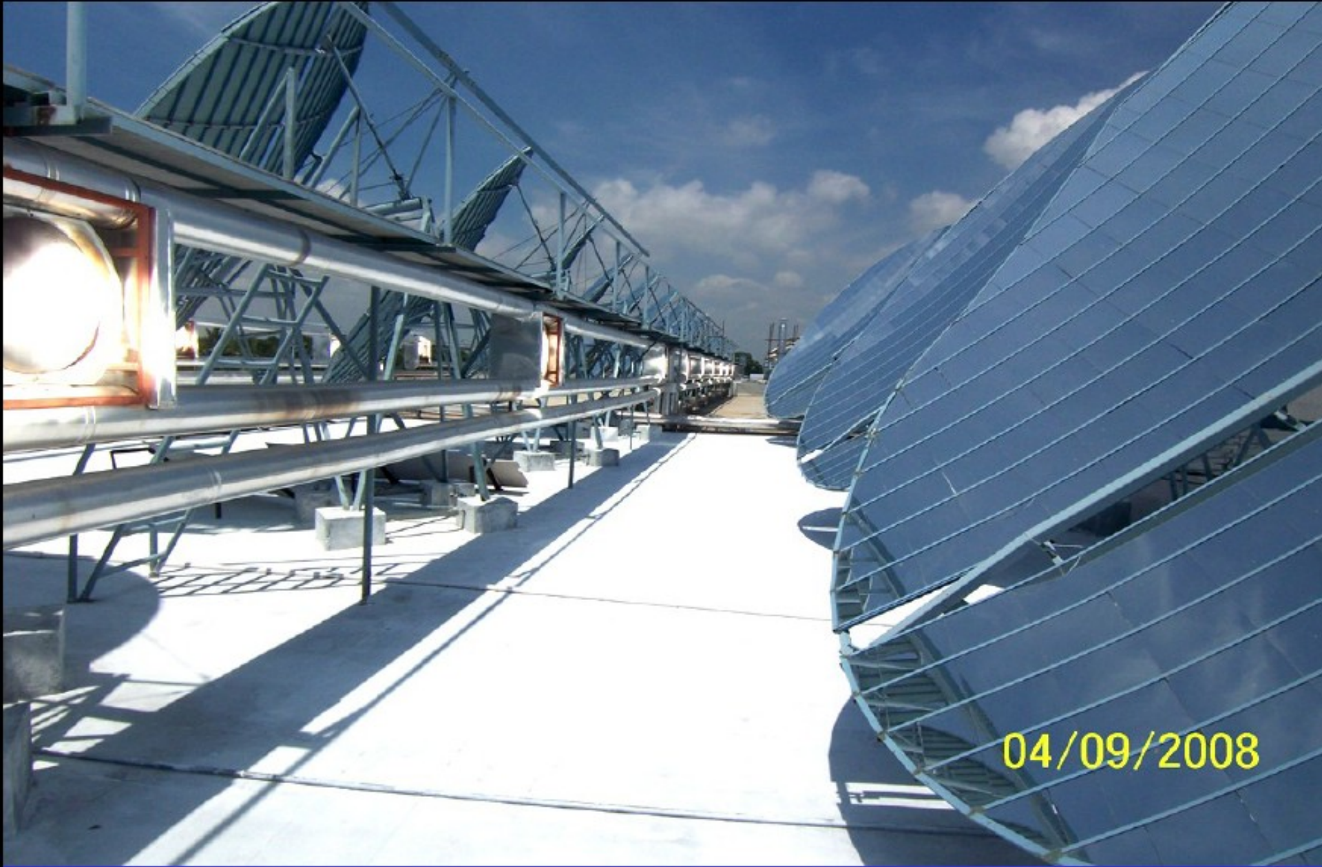
Solar system of 92 TR air-conditioning plant at TVS Suzuki Factory, near Chennai
