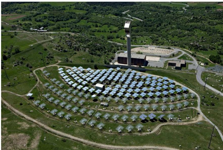
PEGASE Demonstration, 2 MW France, 2016
