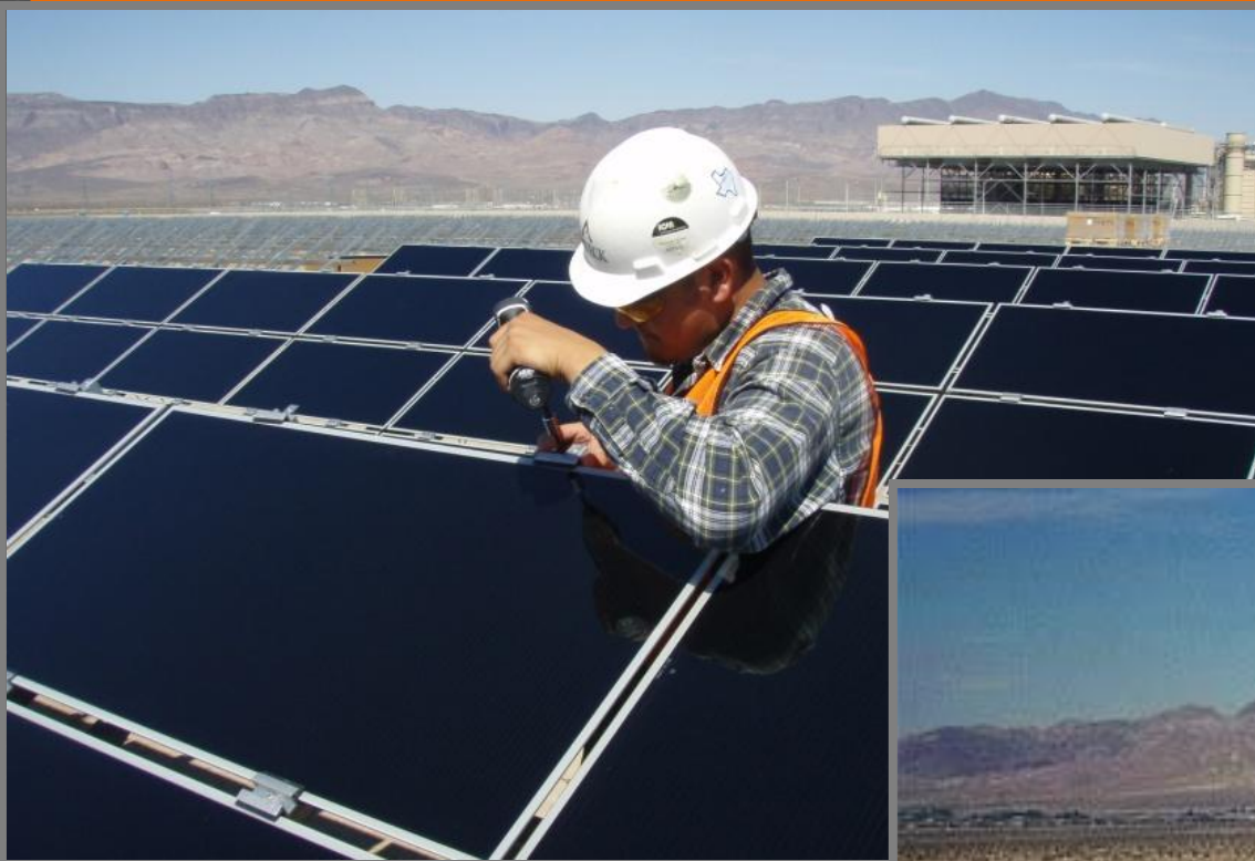
Fixed Tilt Photo Voltaic Panels (PV)
