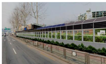
< PV on soundproof walls >
