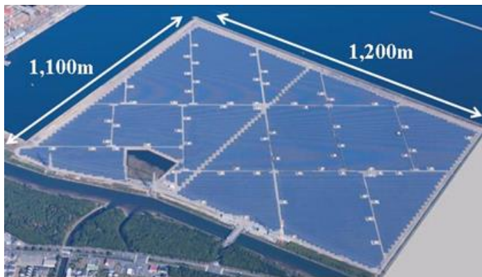
62MW-PV system (Marubeni)
