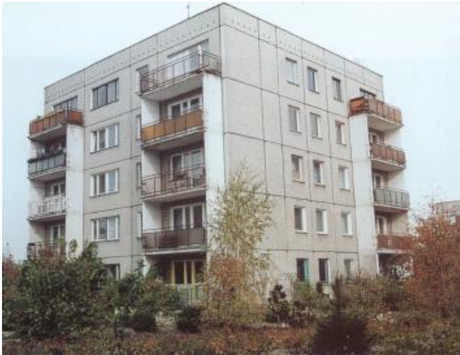
Before thermo-modernisation, Warsaw, 1998
