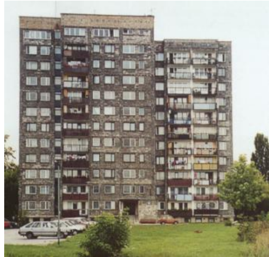
“Eco-buildings” (?) - a fly ash “recycling” technology and application of materials with high radiation for residential buildings
