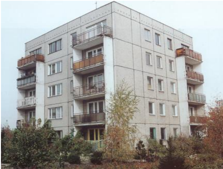
Panel buildings from “building factories” - a Soviet “leading” large panel technology with very poor thermal properties
