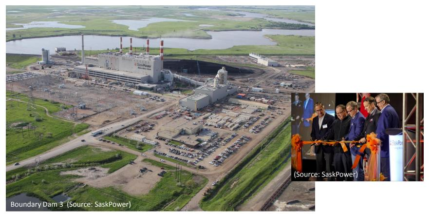
**Size**: 110 MW **Fuel**: lignite **Capture rate**: 90% of CO<sub>2</sub>, **Capture per annum**: 1 million tonnes
