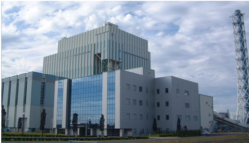
TEPCO Hitachinaka No.1, Japan (Boiler; Babcock-Hitachi ) (600°C/600°C 25MPa 1000MW) (Operation; 2003/12-)
