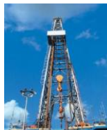
Drilling rig for geothermal power generation
