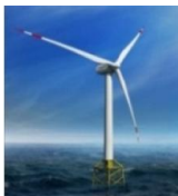
Offshore wind power generation
