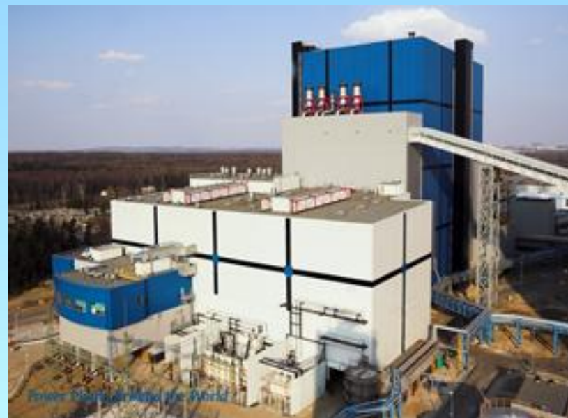
Lagisza 3: 1X 460 MW, the world's first SC CFB power plant
