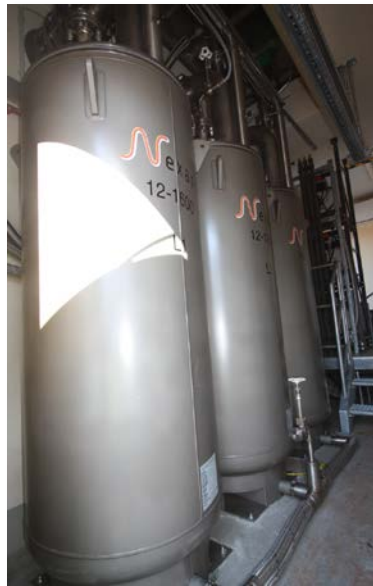
Resistive type, YBCO 12 kV, 1600 A Installed 11/2015
