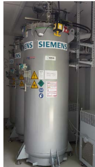
Resistive type, YBCO 12 kV, 815 A Installed 3/2016
