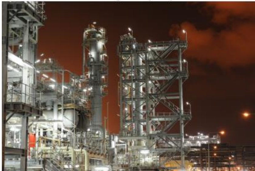
Gas to liquids, Qatar
