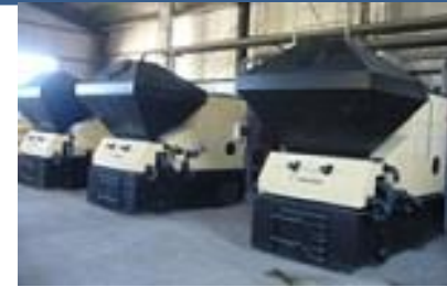
High-efficiency Heat only Boilers, Suuri-Keikaku, Mongolia
