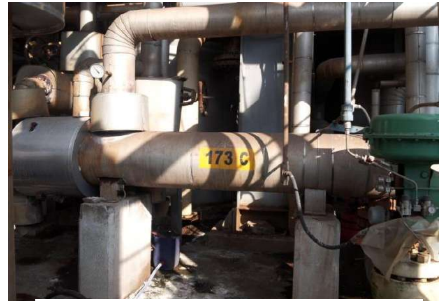
Molecular Sieve Dryer 109-DA/DB
