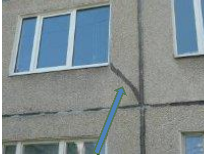
Crushed panel joints
