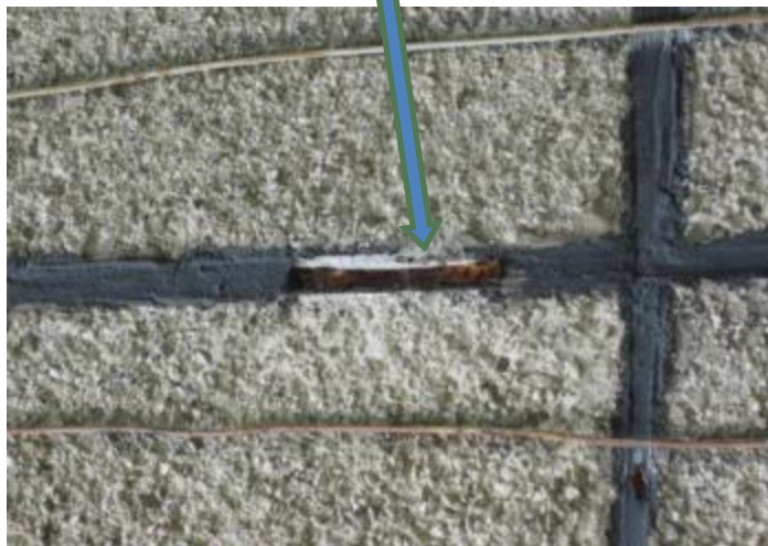
Crushed panel joints
