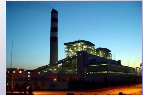
Wangqu - China, 600 MW First SC, 2-pass boiler Chinese lean coal, FGD Cooling tower 40% HHV efficiency
