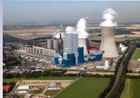
Niederaussem- Germany, 1000 MW SC, High Cr material High moisture lignite, FGD Water cooling NO x control, 37% HHV efficiency
