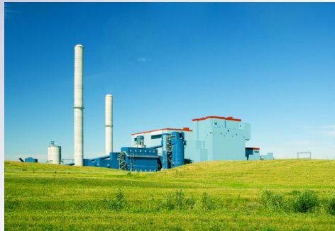
Genesee - Canada, 450 MW SC, Sliding pressure Sub-bituminous coals, SO x & NO x Cooling pond Hg control, 39.6% HHV efficiency
