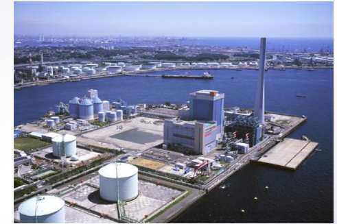
Isogo - Japan, 600 MW USC, High Cr material Bituminous coals, S & SCR Warm sea water cooling Hg control, 40.6% HHV efficiency
