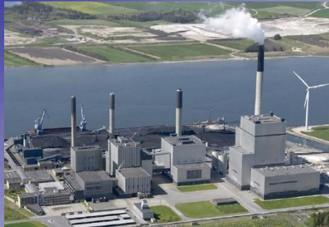
Nordjylland- Denmark, 400 MW USC, innovative cycle design Bituminous coals, FGD, SCR Cold sea water cooling 45.3% HHV efficiency
