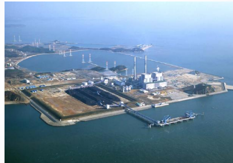
Younghung - Korea, 800 MW SC, tower type boiler bituminous coals, SO x & SCR Warm sea water cooling 39.7% HHV efficiency
