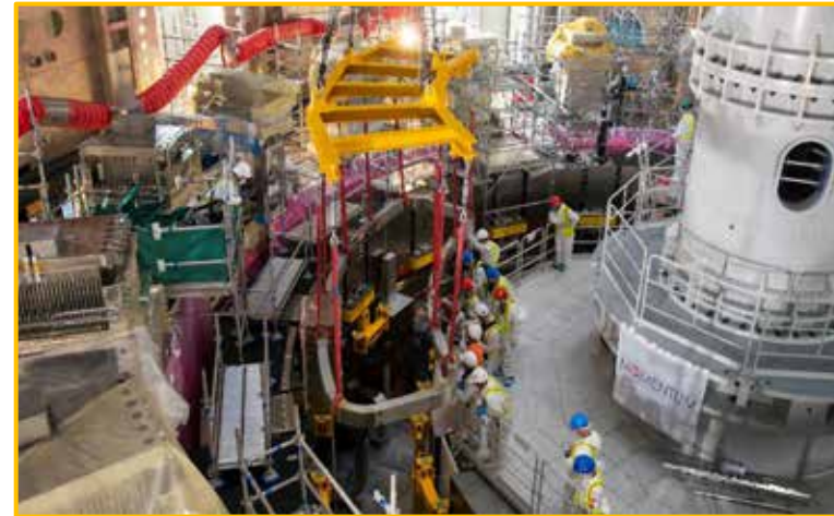
Bottom correction coils installed
