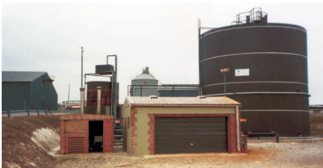
Figure 18 • Anaerobic digestion plant and biogas storage tank
