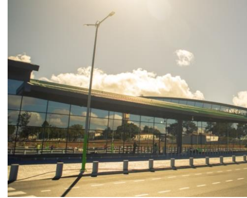
Antananarivo Airport (MDG) Airport by Bouygues and Colas
