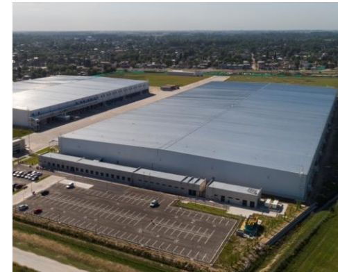
Esteban Echeverria (ARG) Warehouse by Plaza Logistica
