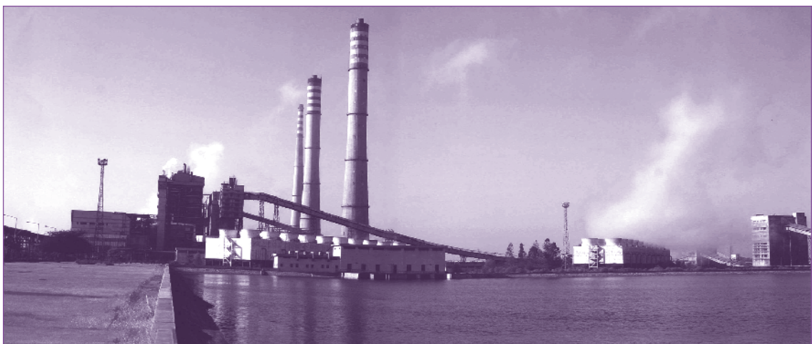
Figure 21 • Suratgarh plant general view
