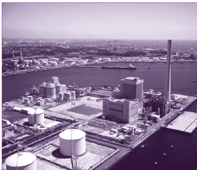
Figure 14 • Isogo New Unit 1 general view
