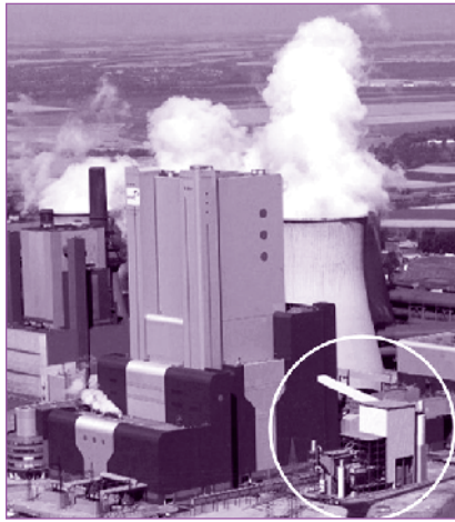
Figure 9 • WTA demonstration lignite drying plant on Niederaussem K
