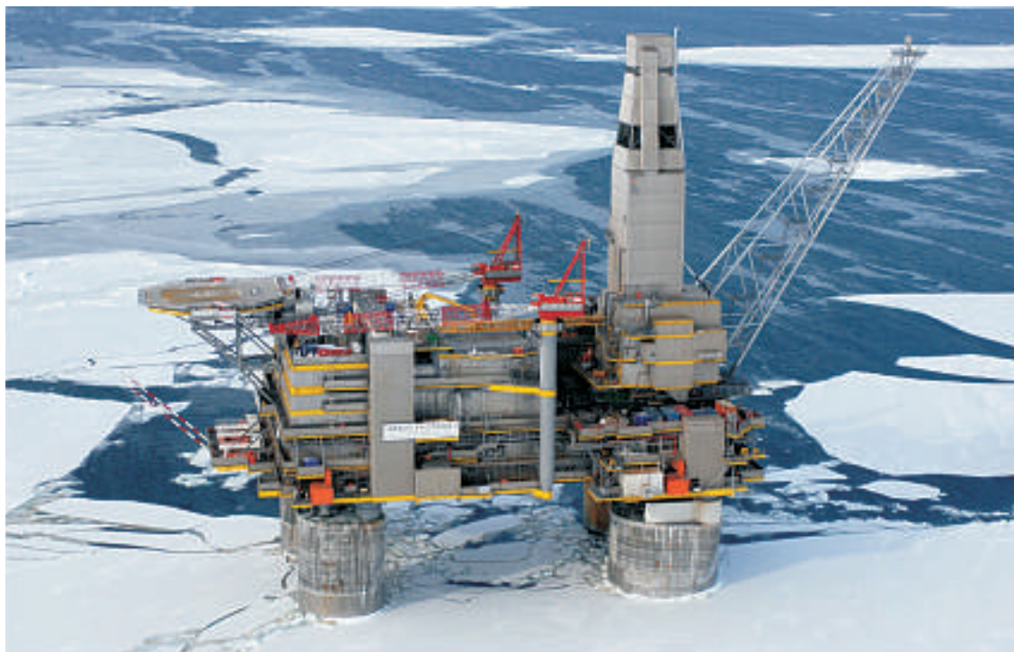
Figure 4.17 • A gravity-based structure to protect against the ice
