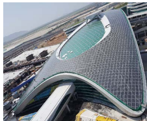
Photovoltaic system installed at Incheon Airport Terminal 2, Incheon, Korea (Photo courtesy of Korea National University of Transportation)
