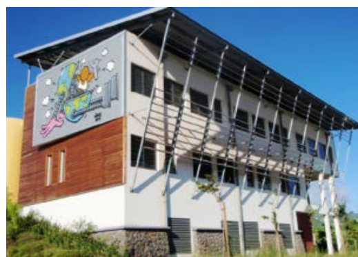
ENERPOS, a net zero energy building in Reunion Island, a tropical climate. (Photo courtesy of Francois Garde)
