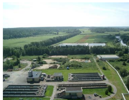
Municipal wastewater plant in Enköping, Sweden, with water storage ponds and (behind the ponds) willow fields that are used as vegetation filters, the harvested willow fuelling an adjacent power plant - (Photo: Pär Aronsson, SLU)
