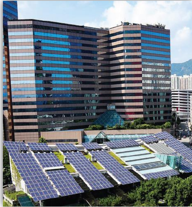
Programme Area No. 4 – Energy Efficiency and Conservation
