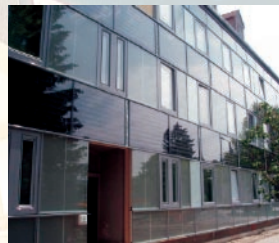
Figure 7: Integration of solar thermal in the building envelop
