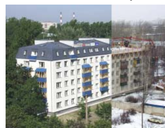
Figure 4: New Roof/storey 17
