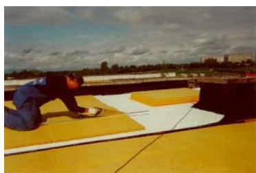
Figure 3: Warm Deck Flat Roof Insulation 16
