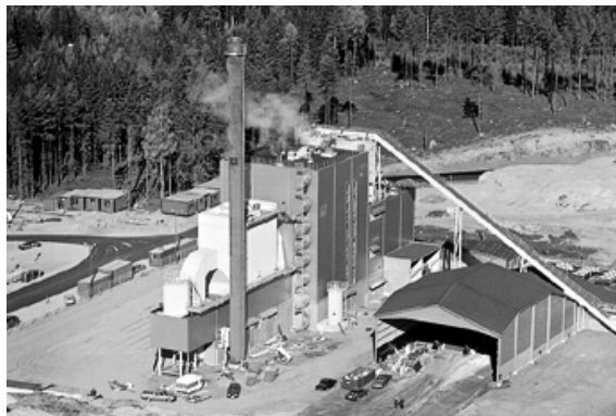
A modern biomass-fuelled power plant at Forssa, Finland
