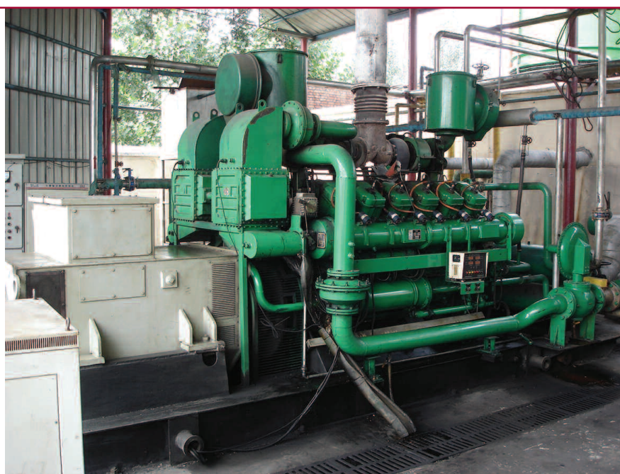
FIGURE 9: LOW GAS QUALITY 500KW SHENGdong ENGINE
