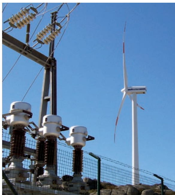
▲ A wind turbine supplying power to the grid.
