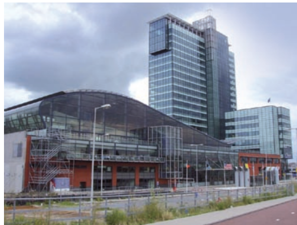
▲ Sustainable heating and cooling in the Oostelijke Handelskade complex (Netherlands).
