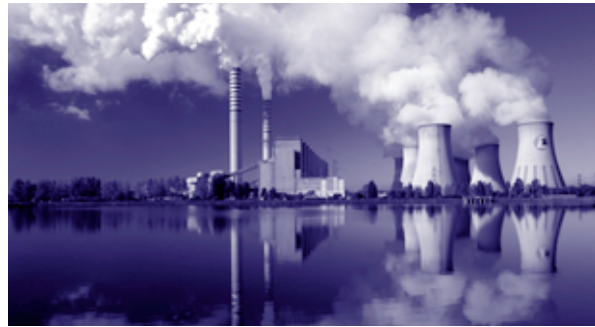
Poland's largest lignite-fired power plant, the 4320 MW Belchatow station, burns 35 Mt/year of lignite.
