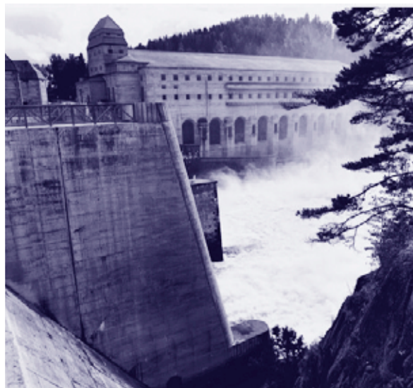
Solbergfoss 110 MW hydro power plant operating since 1924 (Norway).
