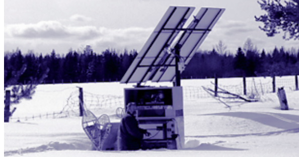
A PV hybrid (PV/propane generator/battery storage) provides electricity to a remote residence (Canada).
