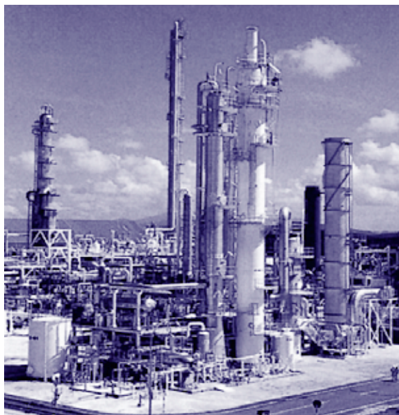
Post-combustion carbon capture at an ammonia plant (Malaysia).
