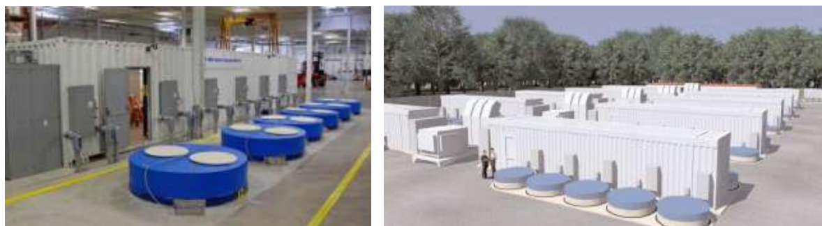
Figure A.49: Matrix flywheel system, showing test facilities at Beacon headquarters (left) and an illustration of the basic concept of a megawatt-scale flywheel-based energy storage system (right).
