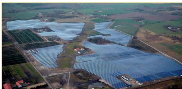
The solar heating plant in Silkeborg is 156 694m 2 and covers 20% of the annual heat demand in Silkeborg, Denmark. (Source: Silkeborg Forsyning A/S).
