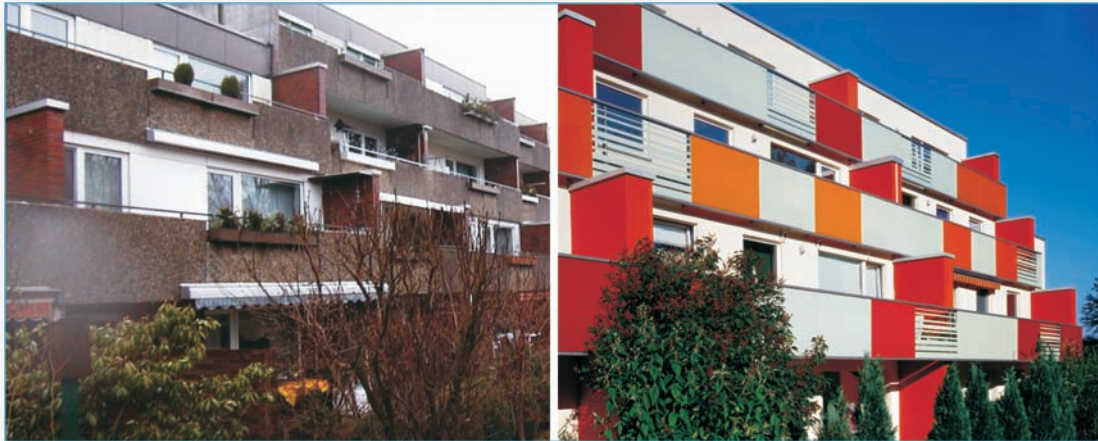
Figure 3.11 Wall retrofit for energy efficiency with EIFS
